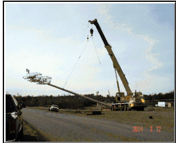
Installing Booneville Football Field Lights
