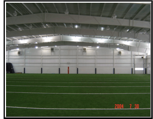
Greenwood Multi-Purpose Facility
