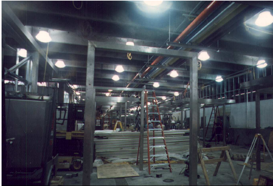
Figure 3 - Plant Interior During Construction
